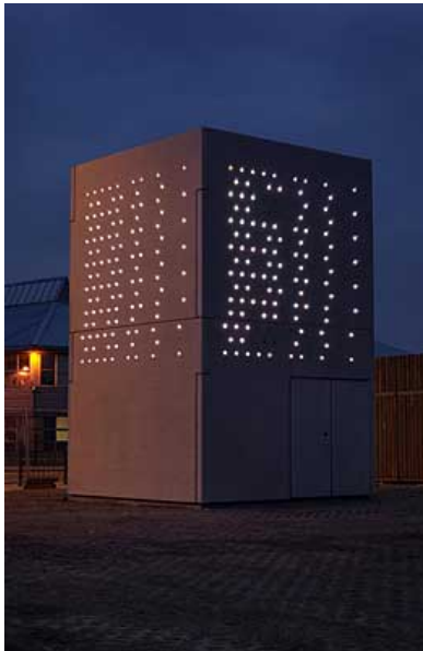
Pump House, designed by Tom De Paor and lighting artist Clare Brew
